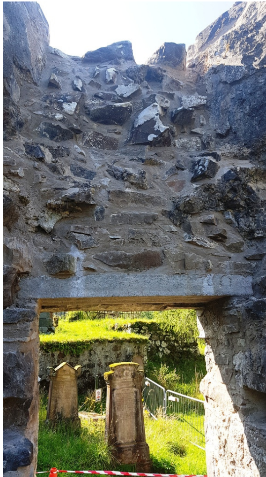
Concrete lintols below inner face
