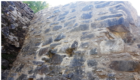
Joist dooks either side of opening internal face
