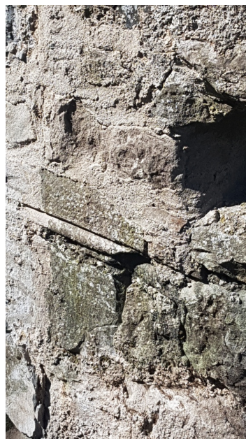
Evidence of window opening before creation of door
