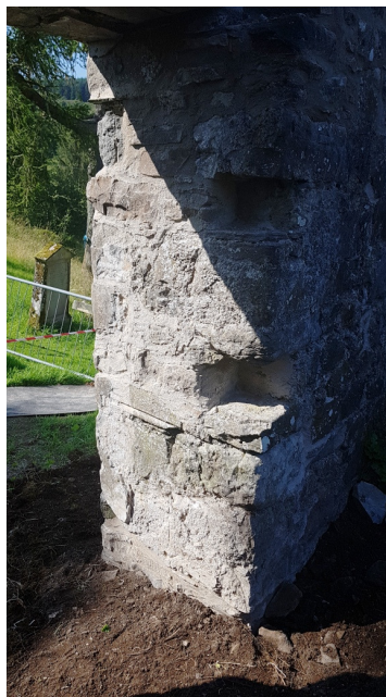
Evidence of window opening before creation of door
