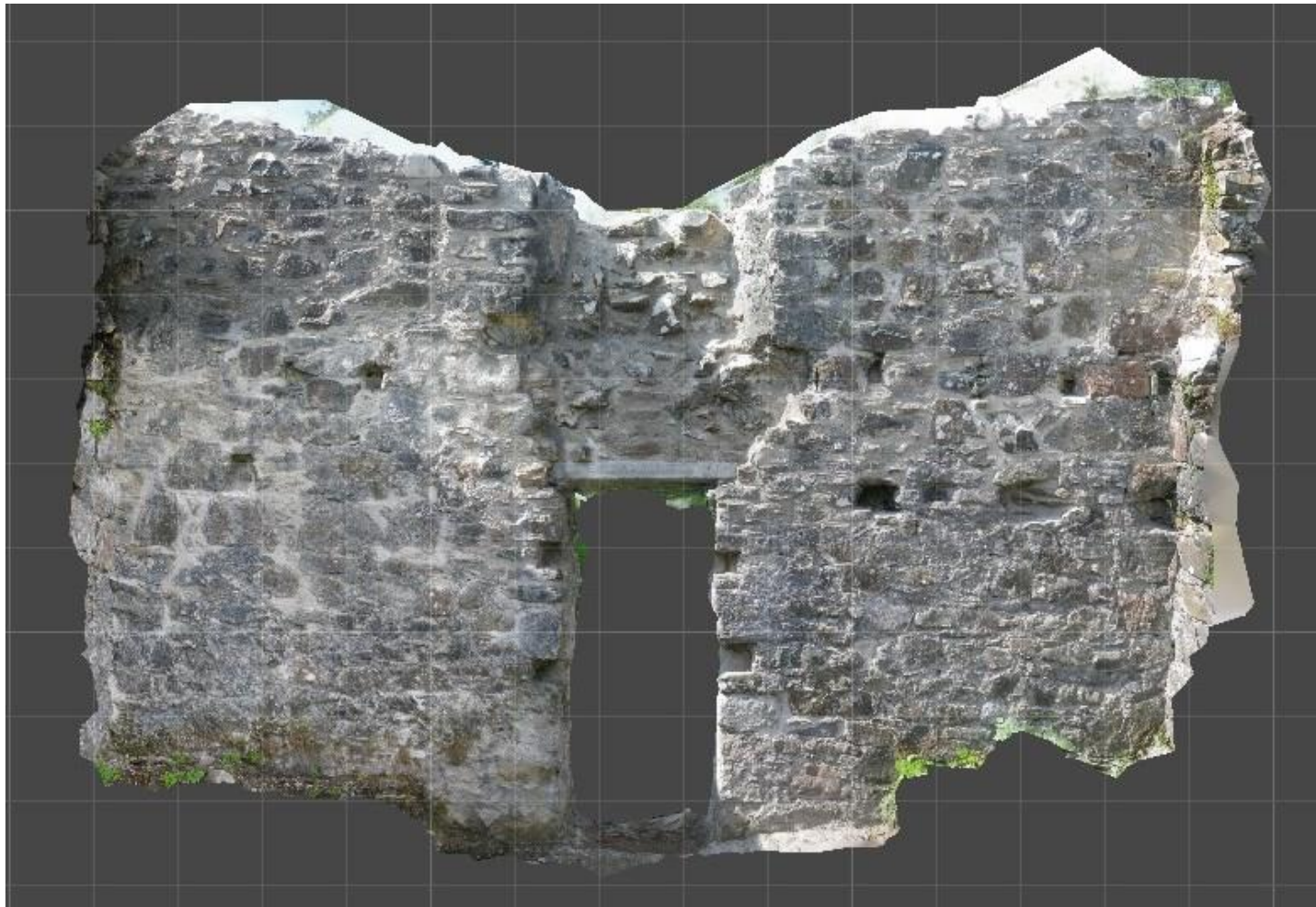
Fig. 3. The internal elevation following the consolidation works and prior to backfilling of Trench 1.
